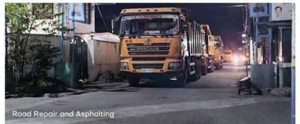
Road Repair and Asphalting
